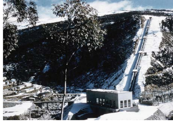
Guthega power station 60 MW
