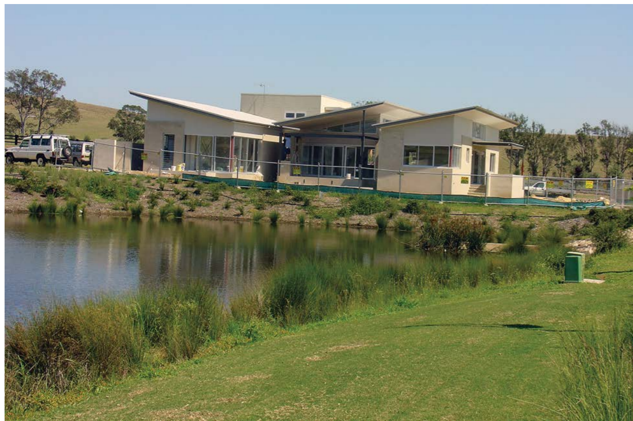
Vintage house under construction
