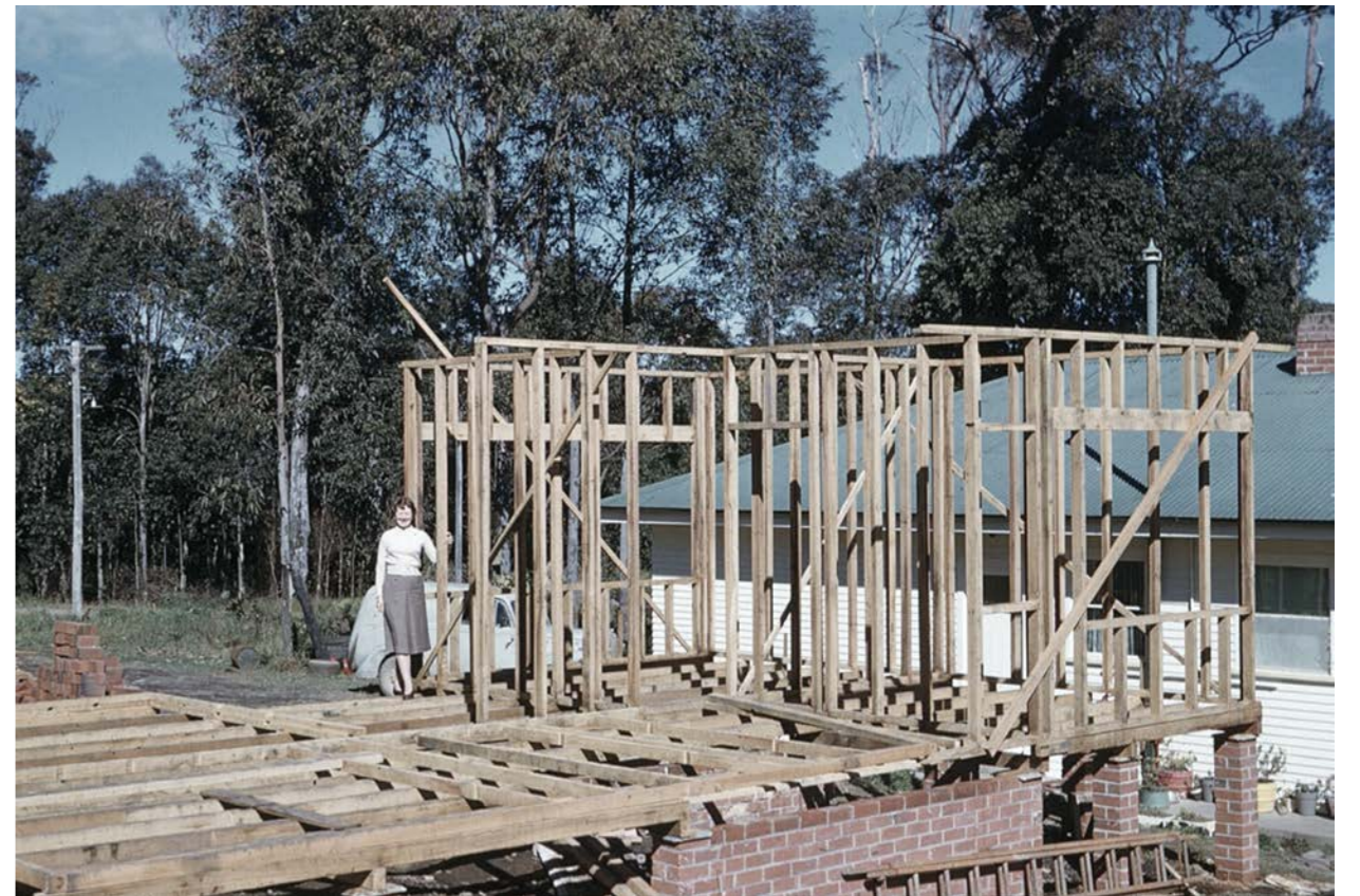
Nan inspecting construction
